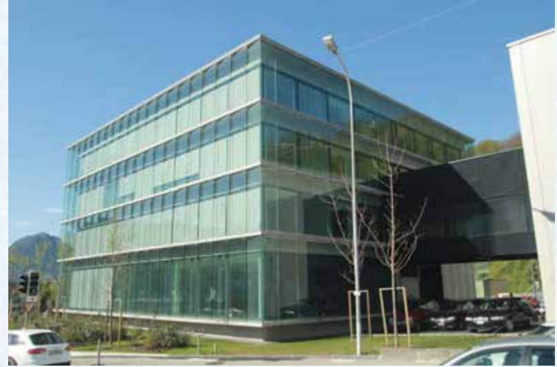
700 kW energy consumption, cooling with 700 l/s water from Lake Lugano
