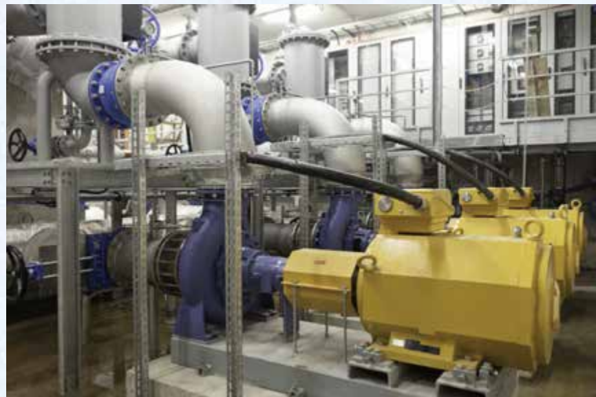
700 kW energy consumption, cooling with 700 l/s water from Lake Lugano
