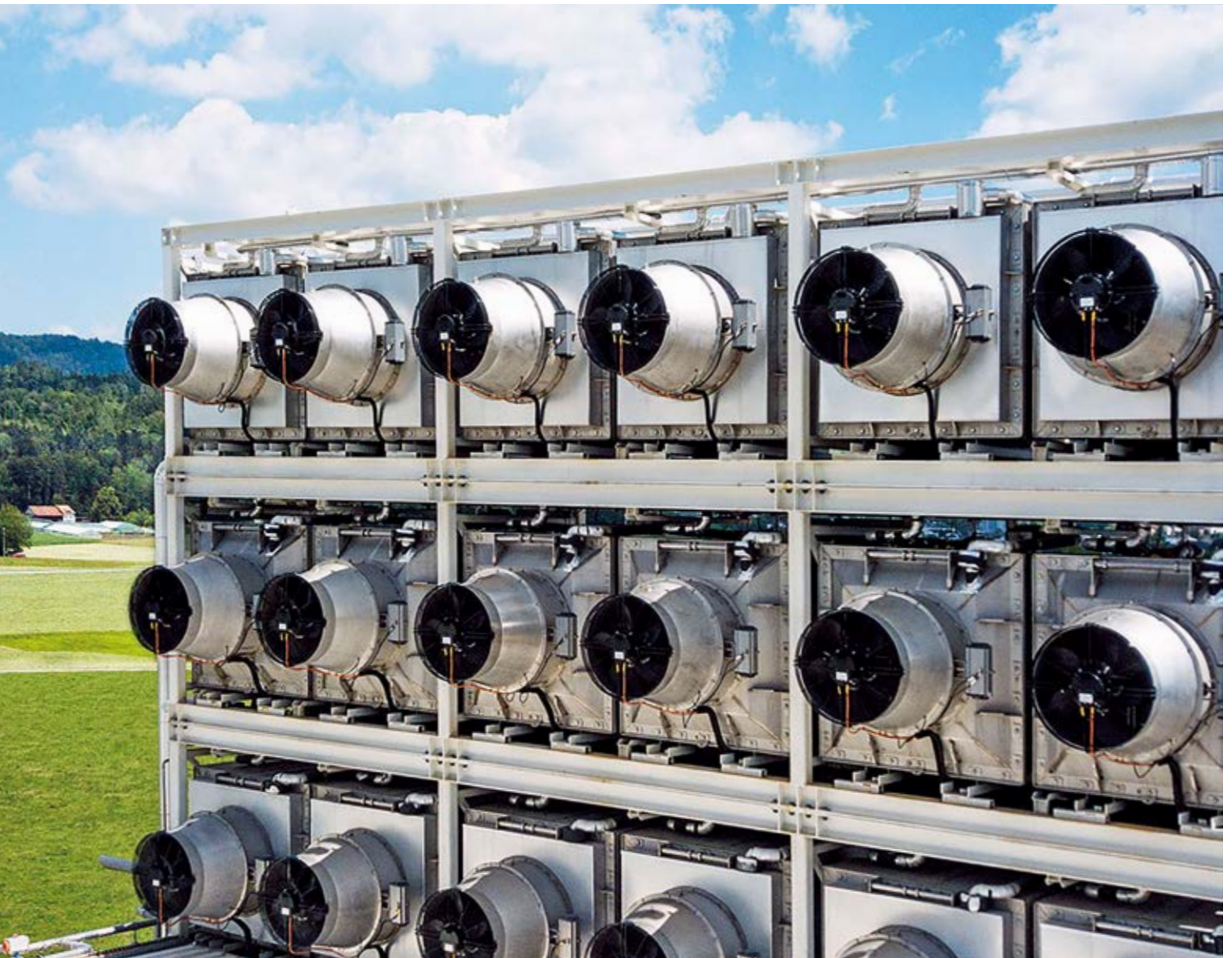
Using the technology developed at ETH by Climeworks, excess carbon dioxide is filtered out of the atmosphere. ETH spin-off Climeworks is a so called unicorn, i.e. a start-up with a market valuation in excess of CHF 1 billion. (Image: Climeworks)
