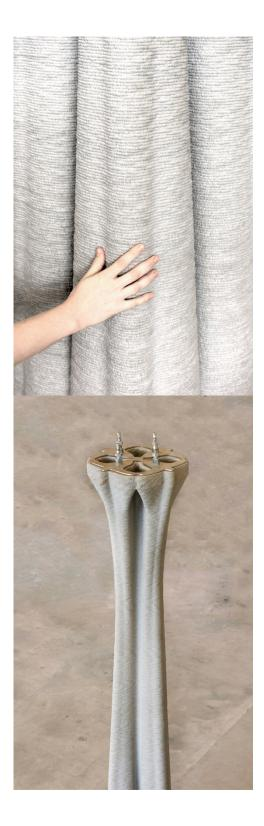
Concrete textured surface of a Concrete 3D Printed Colum, Scientifica 2019: Science Fiction Science Fact © Axel Crettenand, Digital Building Technologies ETH Zurich
