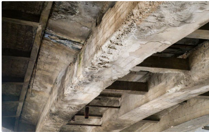
Corrosion is a gradual process that often remains unnoticed until it's too late. This image shows the degraded substructure of a steel-reinforced concrete bridge.
