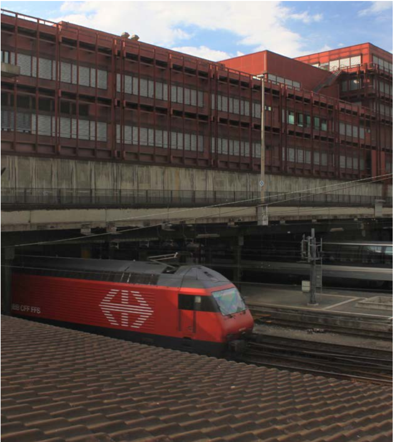
Peter- Merian Brücke Basel, 2013
