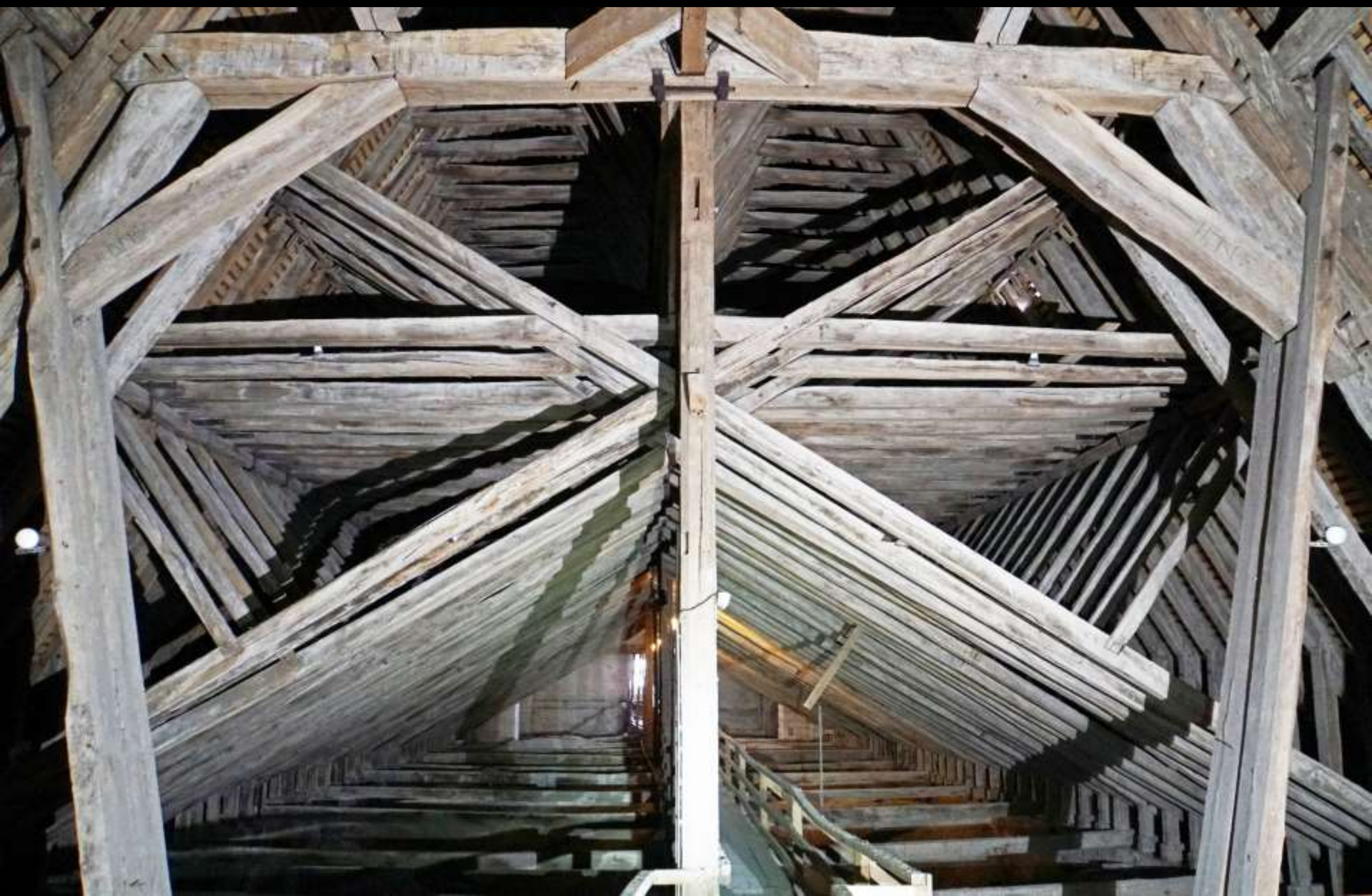
Sens, Kathedrale, Langhaus, Dach (1267d – 1293d)
