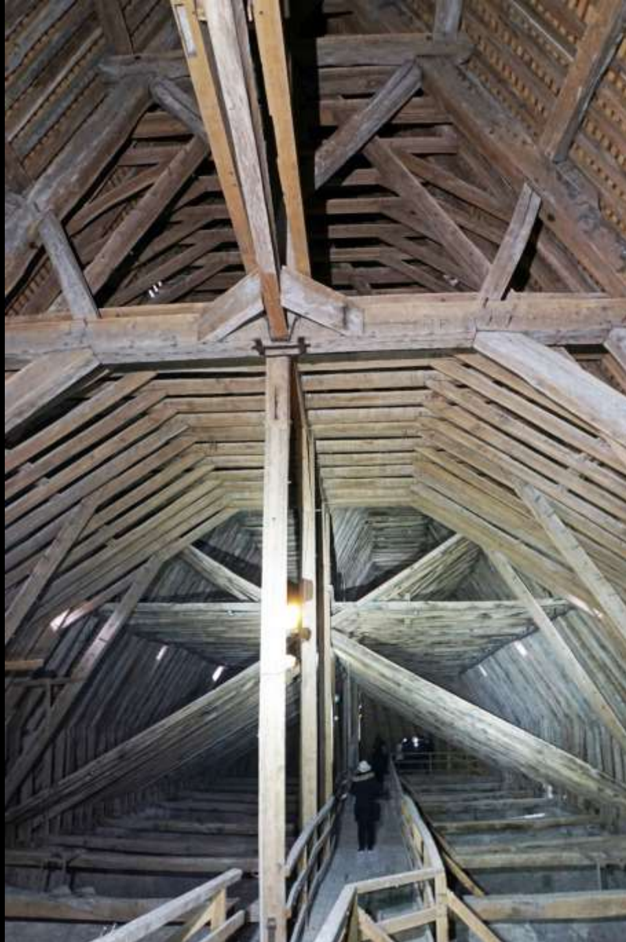
Sens, Kathedrale, Chor, Dach
