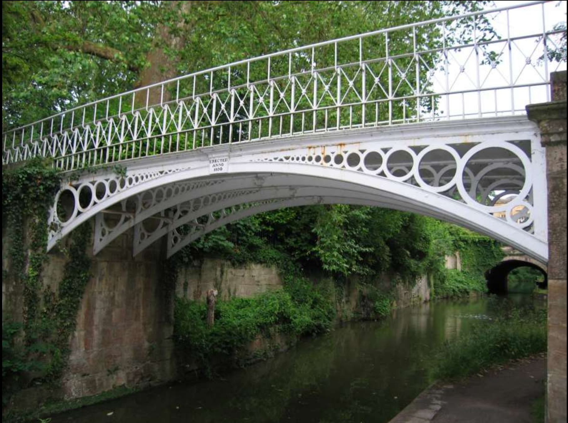
Bath, Gusseisen-Brücke in den Sydney House Gardens (1800)
