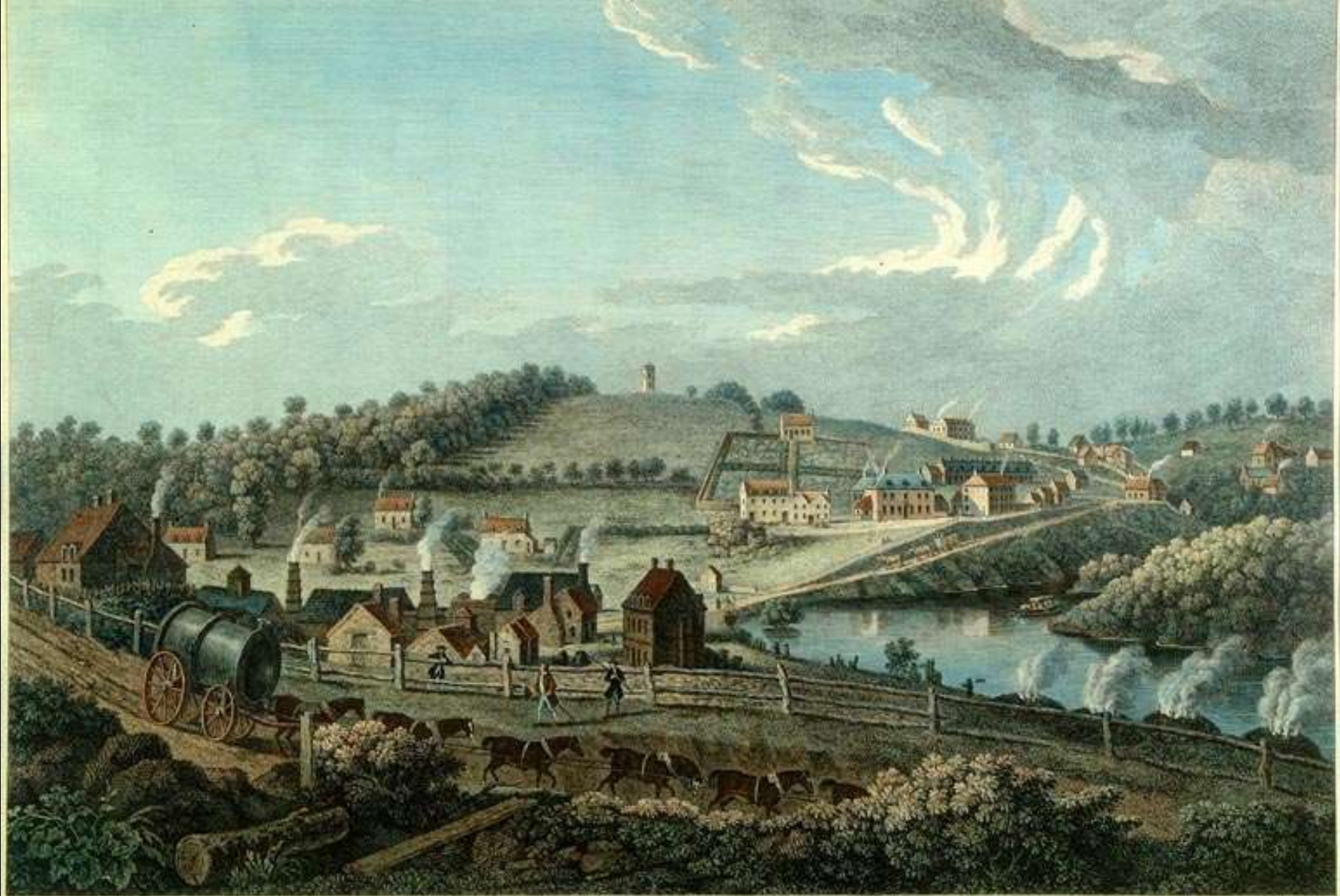
A VIEW of the Upper Works at Coalbrook-Dale, in the County of SALOP. T. Smith 1758 according to the Original. Designed and Engraved by G. Perry and
