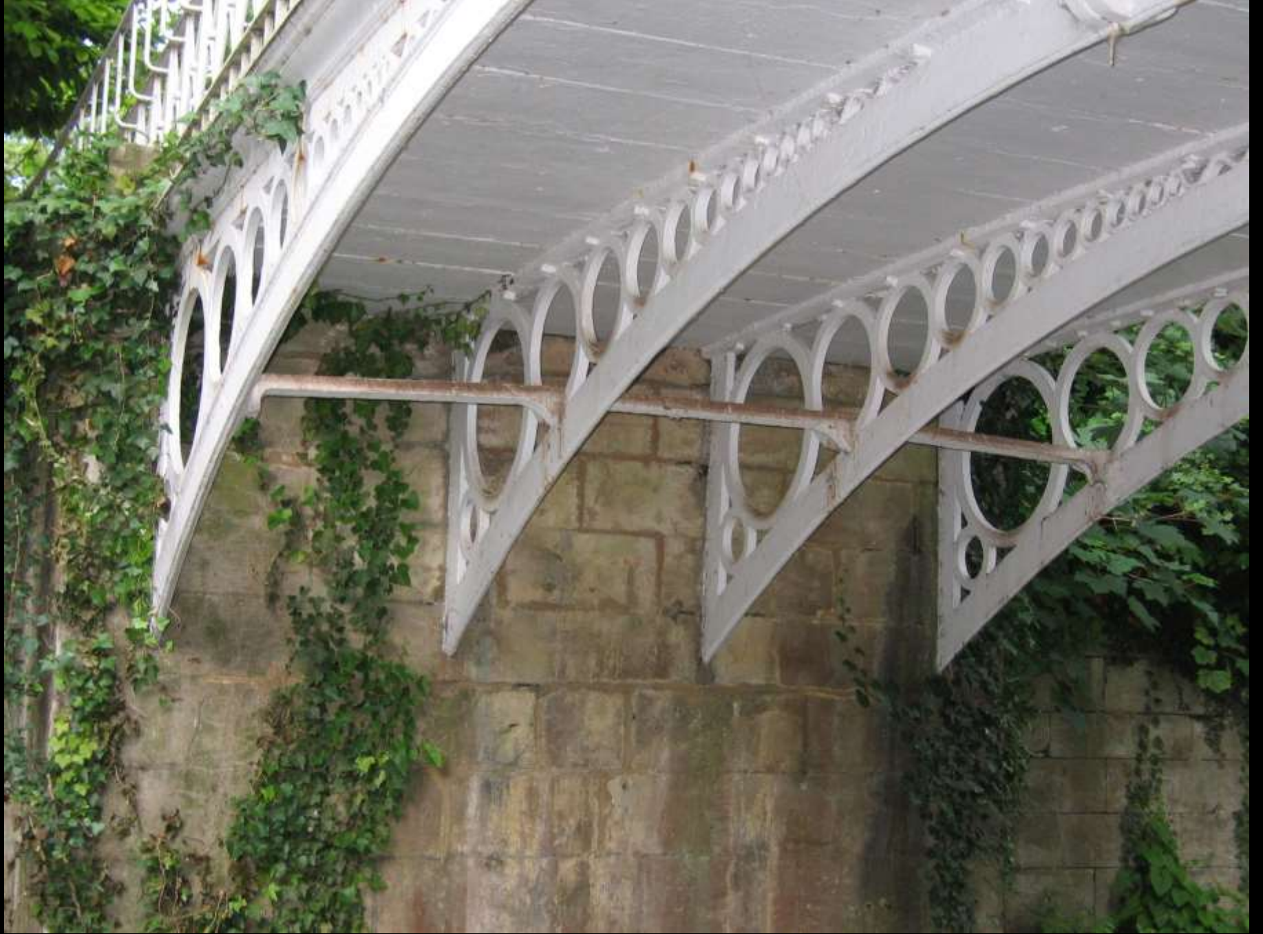
Bath, Gusseisen-Brücke in den Sydney House Gardens (1800)
