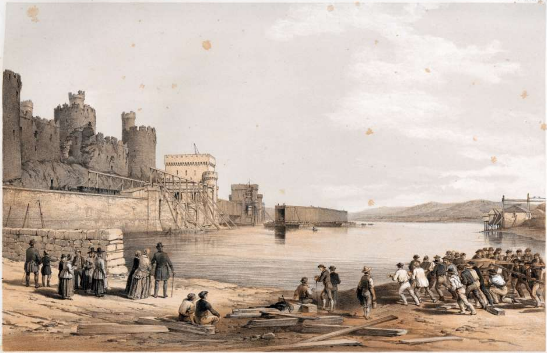
CONWAY BRIDGE. GENERAL BRIDGES, GREAT BRITAIN.
