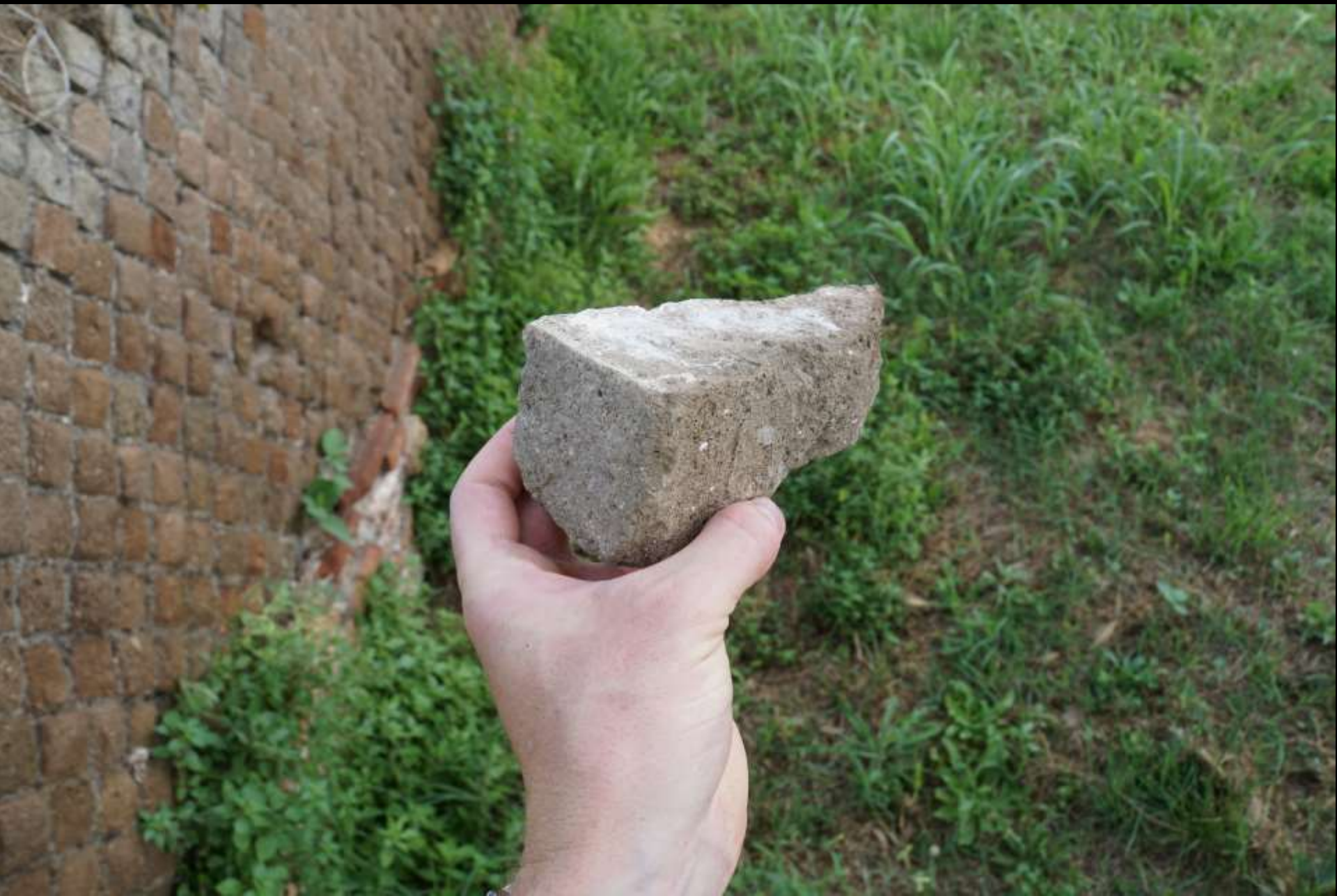
Opus reticulatum, Detail (Ostia, Foto: W. Potgeter)
