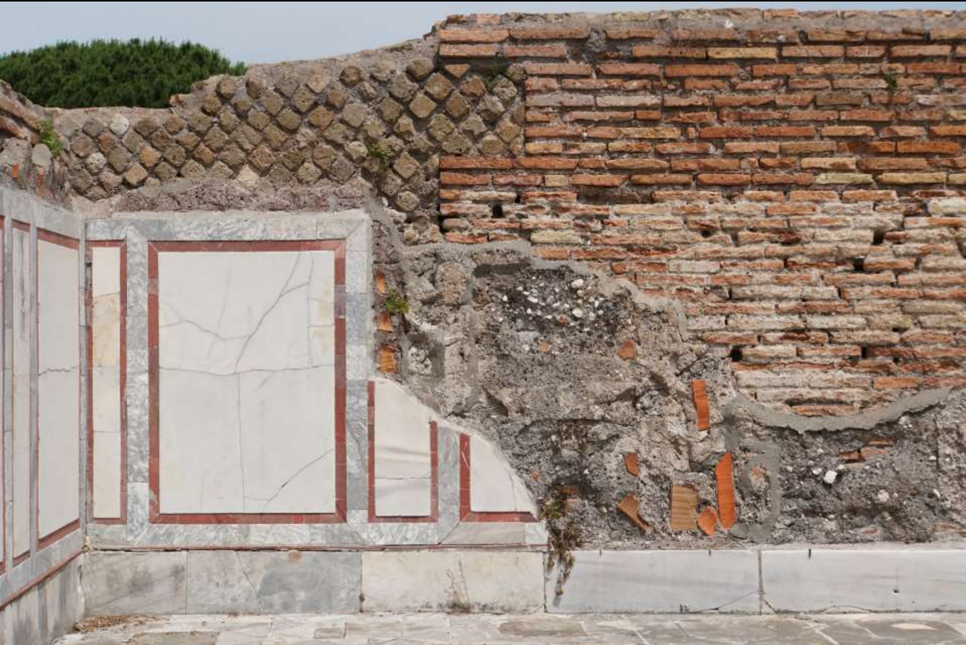
Buntmarmor-Intarsien ( opus sectile ) (Ostia; Foto: W. Potgeter)
