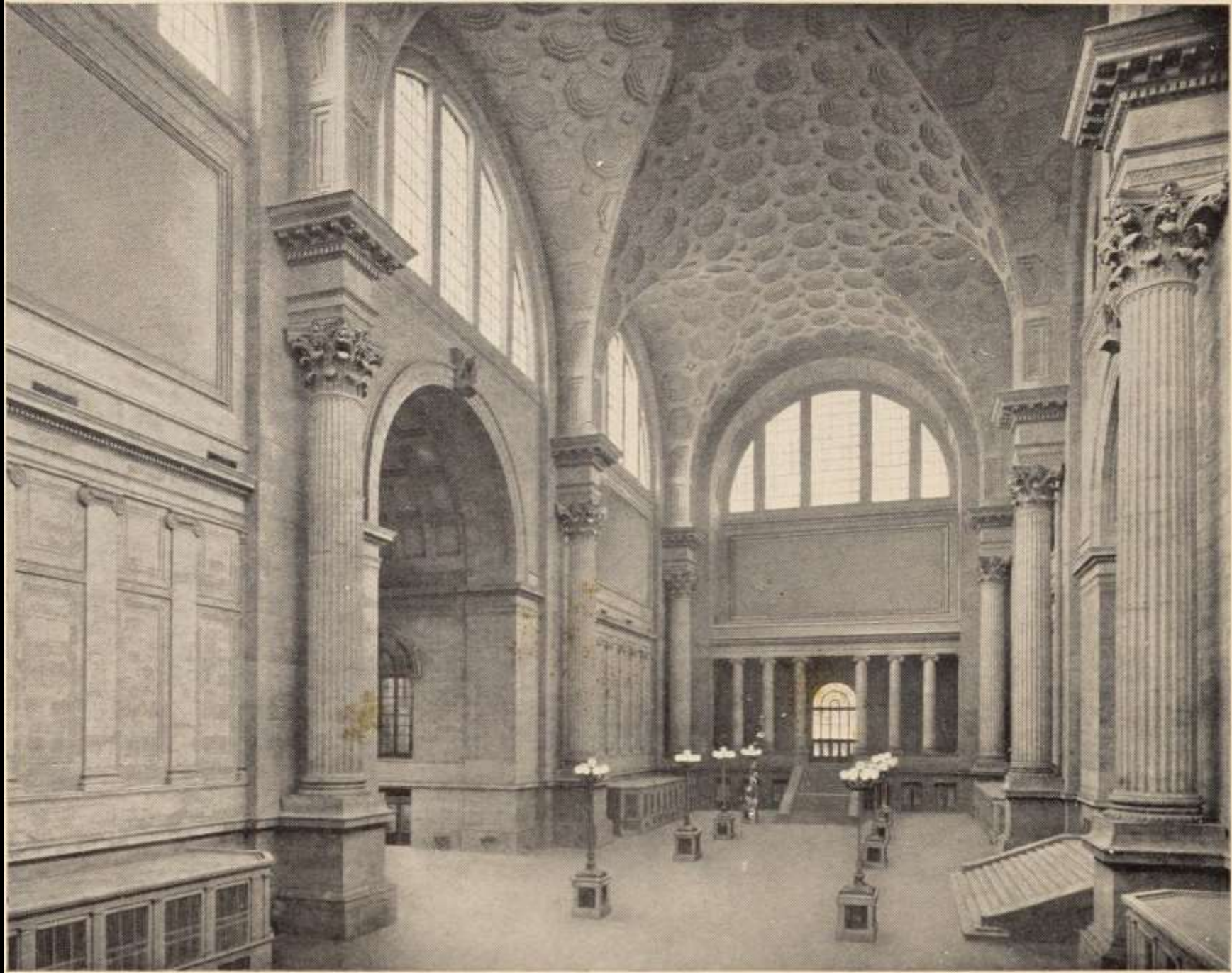
New York, Pennsylvania Station, Hauptwartesaal (1910; Library of Congress)
