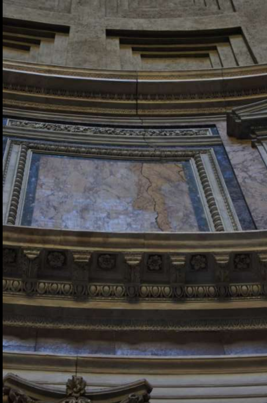
Rom, Pantheon. Kuppel. Riss in der Attikazone
