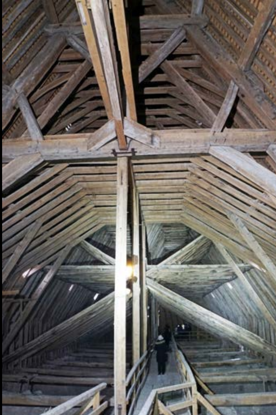
Sens, Kathedrale, Chor, Dach
