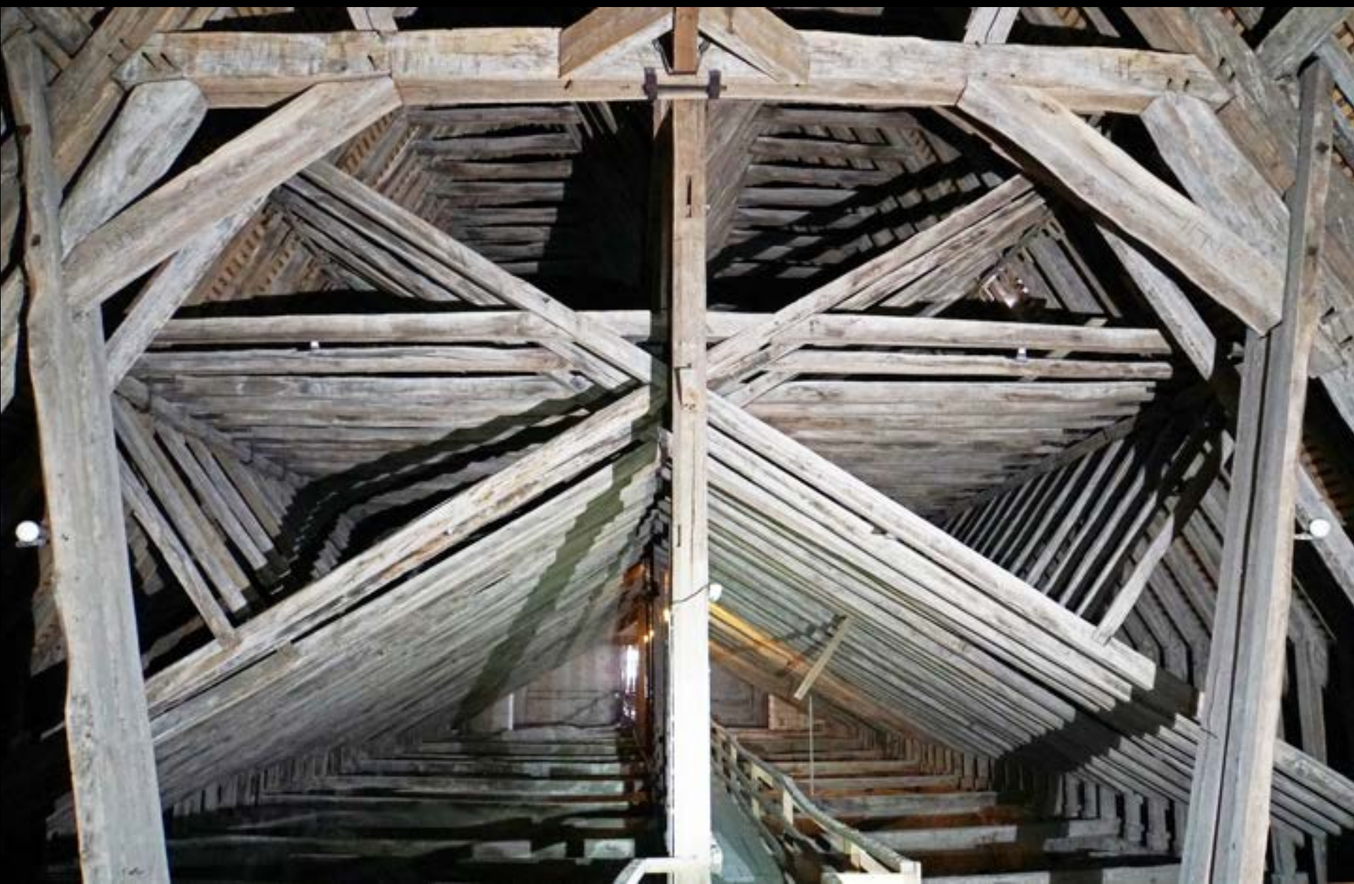
Sens, Kathedrale, Langhaus, Dach (1267d – 1293d)
