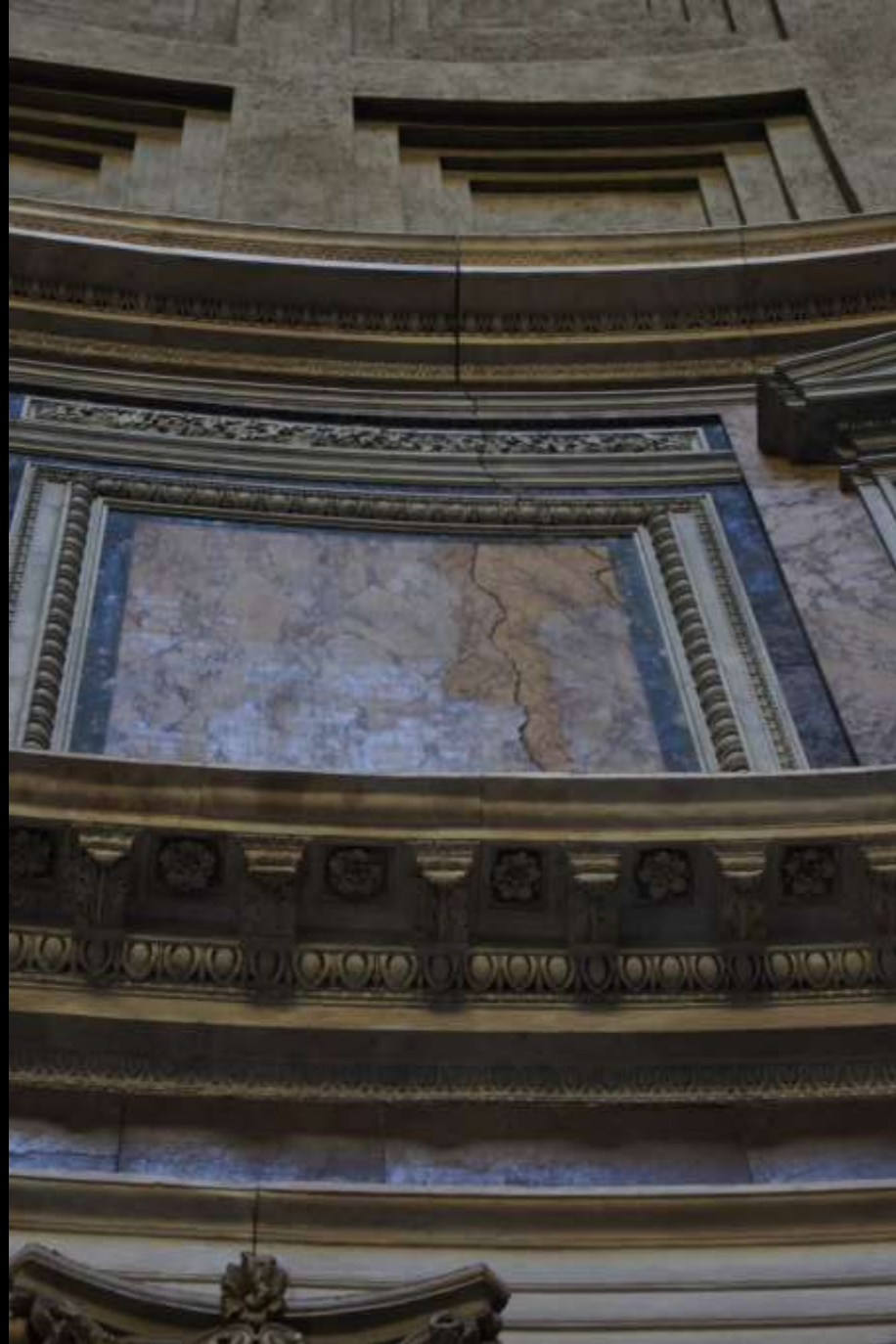
Rom, Pantheon. Kuppel. Riss in der Attikazone
