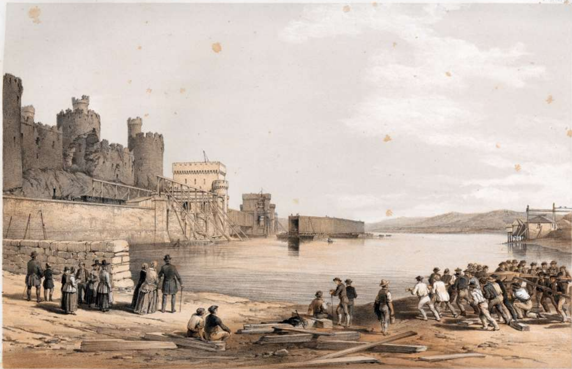
CONWAY BRIDGE. GENERAL BRIDGE, TRAIL, LOWER BRIDGE.
