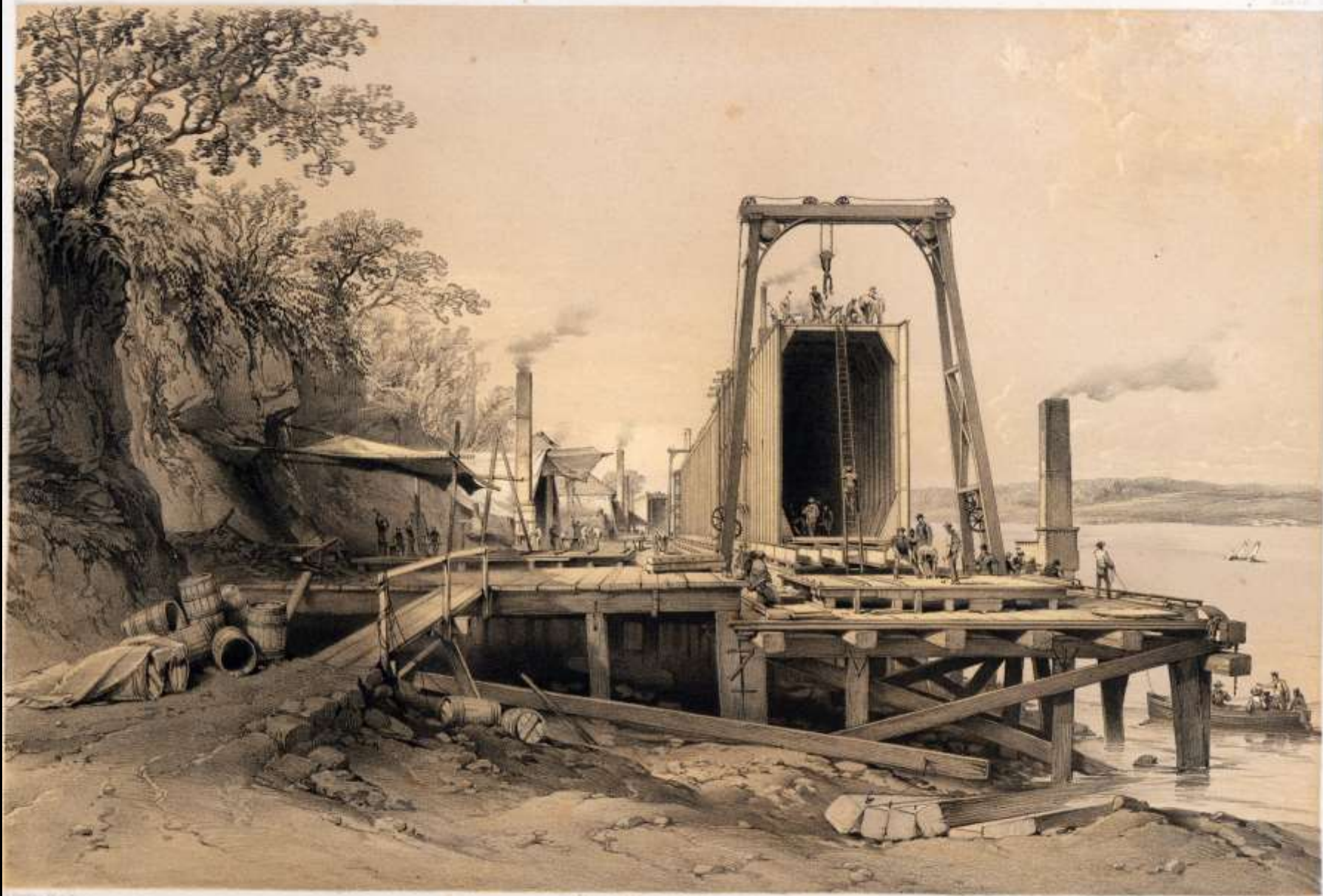
BRITANNIA BRIDGE. PLATE I. THE TRUSS IN POSITION ON THE PIER, SEPTEMBER, 1850.
