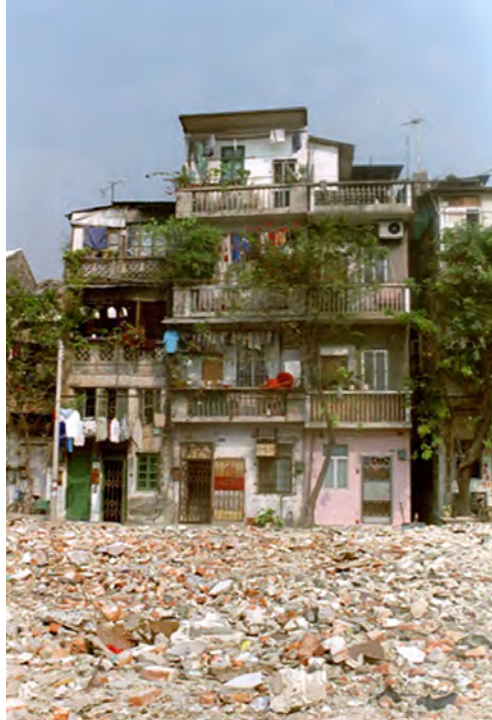
Fig. 5) Waiting for the bulldozer
