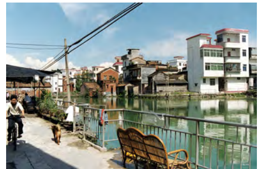
Fig. 15) New 4-storey houses “disturb” the building structure of the old village parts
