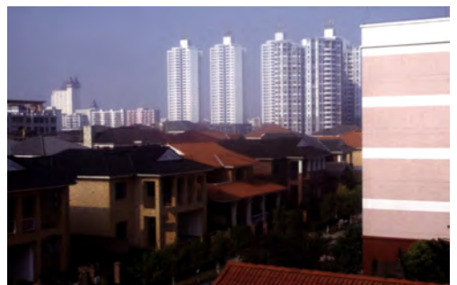
Fig. 8) Riverside Garden highrises and villas, new housing for 50'000 upper middle class people
