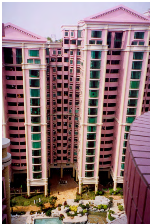
Fig. 7) Post modern condominiums with penthouse apartments sold for 500'000 US $
