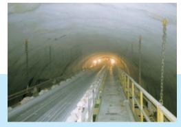
Suspended infrastructure platform for the blasting work: NEAT, Loetschberg axis, Mitholz face.
