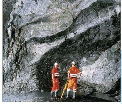
Intensively folded sedimentary rock at the depth of 1200 m at Ferden (Lötschberg base tunnel)
