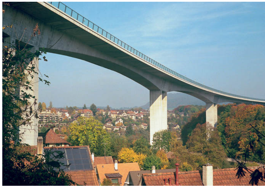
Fig. 2: Balanced cantilever spans.
