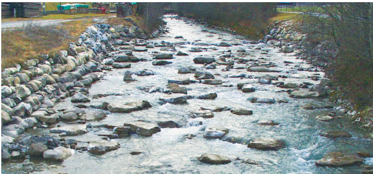
Fig. 47: Unstructured block ramp in the Simme river near St. Stephan (Kt. Berne).
