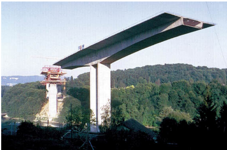
Fig. 5: Balanced cantilever construction.
