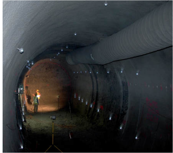
Fig. 2: View from the total station console: The prisms are ordered in profiles approximately 1.5 m apart. The total station was used for tunnelling and the heading face. In addition to the geodetic and geotechnical measurements geologists were mapping the surface of the tunnel every evening.
