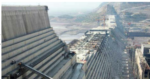
The construction of the Grand Ethiopian Renaissance Dam on the Blue Nile River at the end of 2017. The dam provoked tensions between Ethiopia and its neighbours – echoing the situation following construction of Gibe III mega-dam on the Omo River.
