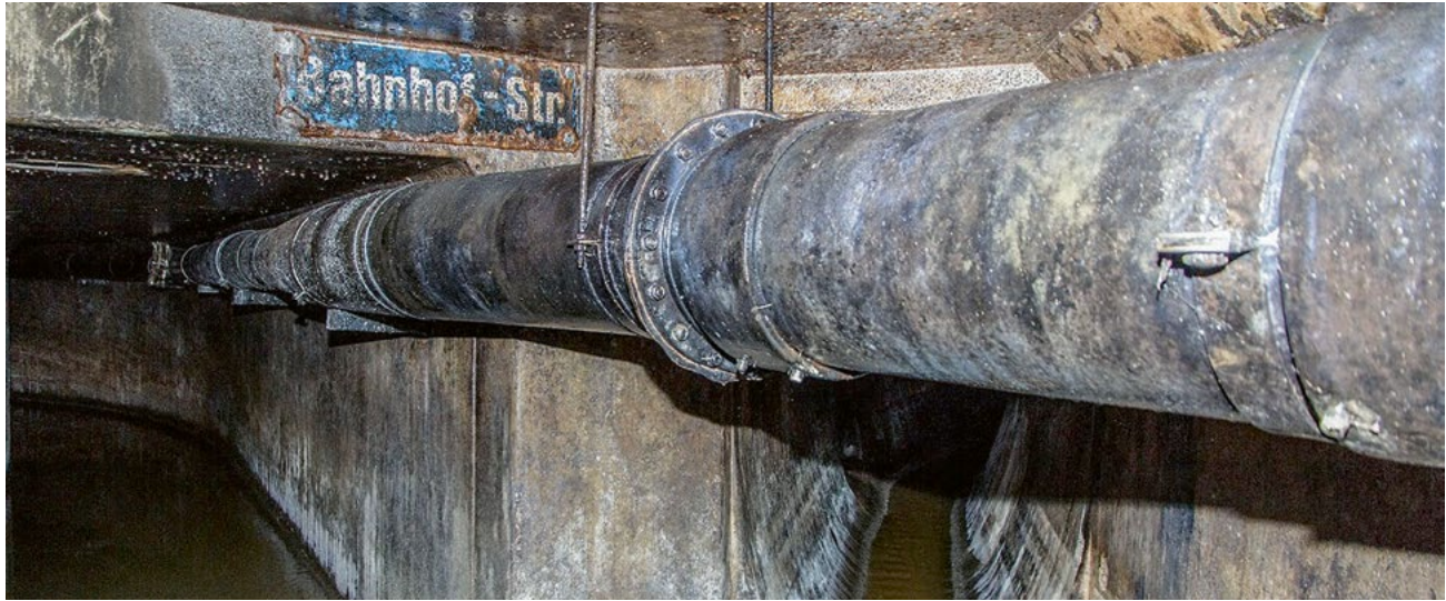
📍 Beneath the Bahnhofstrasse in Zurich, a sewer conveys wastewater to the treatment plant. Rainwater is channelled through a separate pipe.
