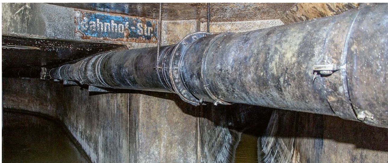
↑ Beneath the Bahnhofstrasse in Zurich, a sewer conveys wastewater to the treatment plant. Rainwater is channelled through a separate pipe.
