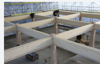
Construction of the pre-stressed timber frame
