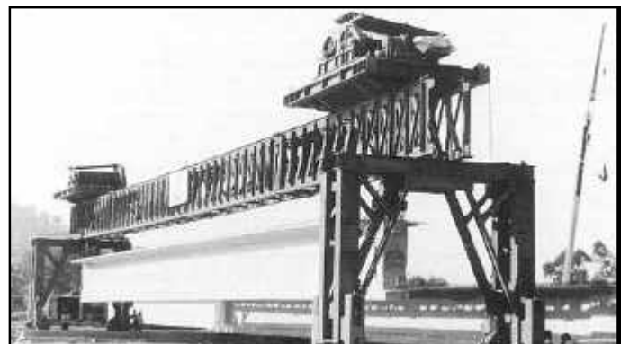
Figure 5.3.2: Modified T-beams replaced the originally designed I-beams and eliminated the deck slab formwork.
