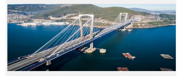
The Atlantic Motorway, AP-9, crosses the Vigo estuary by means of a 400 m span cable-stayed bridge over the Rande Strait. This bridge was built between 1973 and 1977, and opened to traffic in 1981. In 2006, the average daily traffic reached 47 000 vehicles, close to its effective capacity and therefore resulted in frequent traffic congestion conditions.
