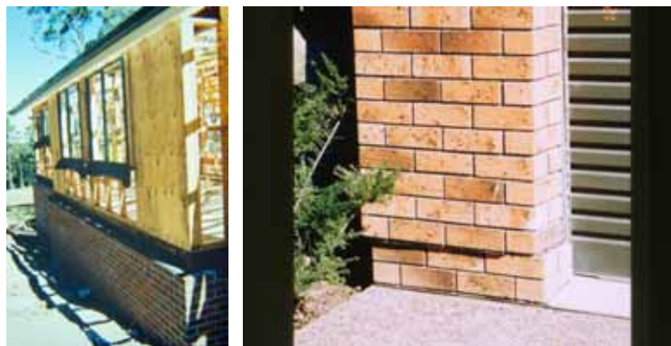
Figure 1: Typical DPC practice and earthquake performance
