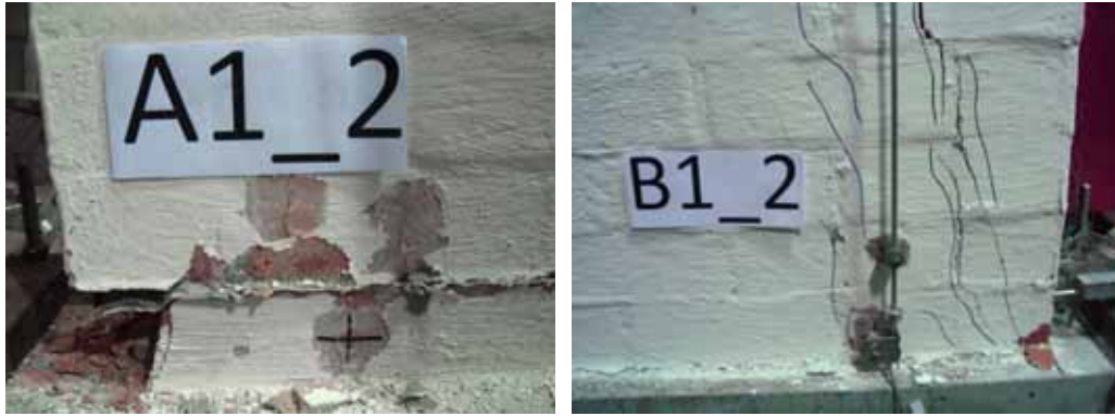
Figure 28: Failure of the specimens A1_2 and B1_2
