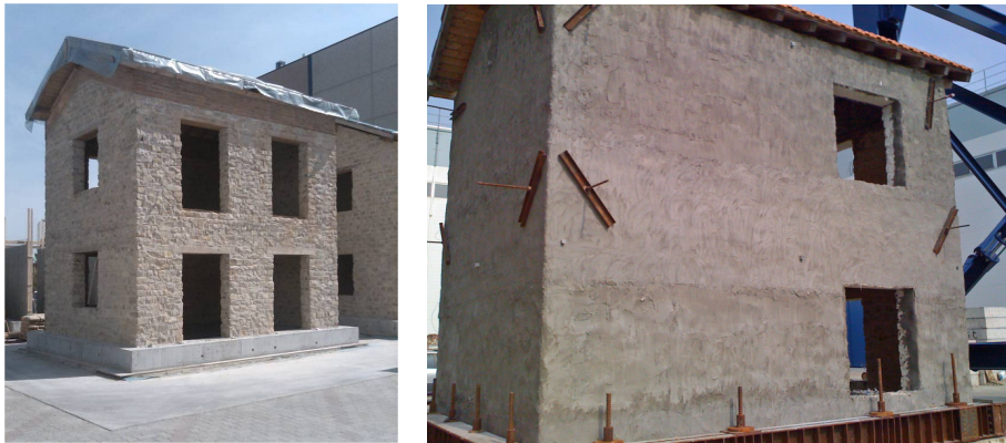
Fig. 5: 3D View of the unreinforced (left) and reinforced (right) stone building, reproduced from [66, 17].
