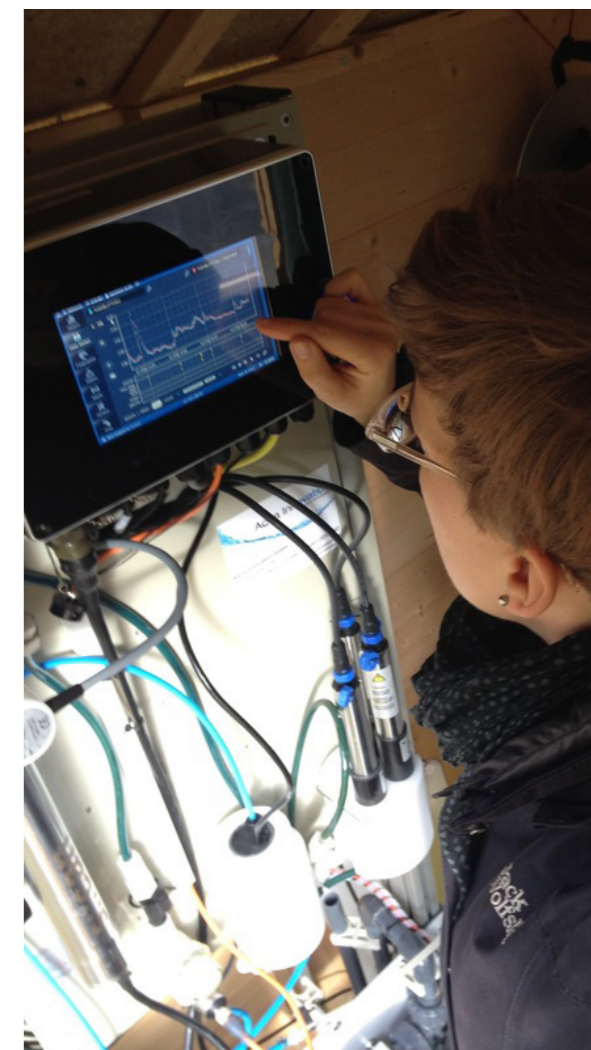
Checking the real-time monitoring of water quality. Credit: J. von Freyberg.
