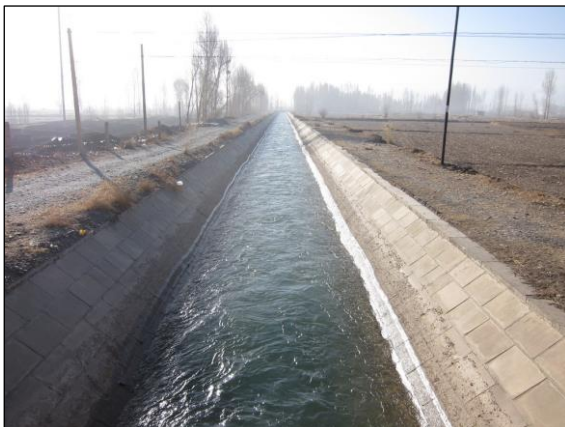
Figure 47: Second order irrigation channel
