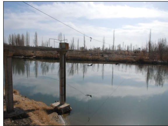
Figure 4: Heihe River middle section: Gaoya flow measurement station
