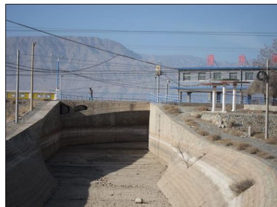
Figure 50: East main channel diversion
