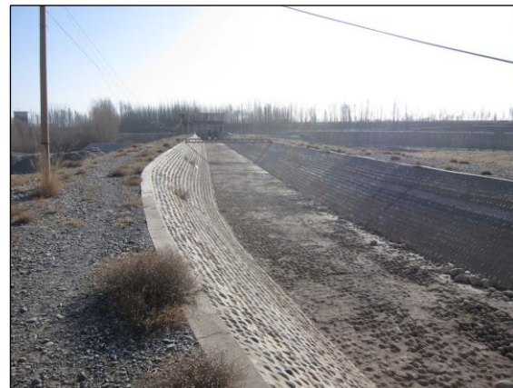
Figure 48: First section of the east main channel
