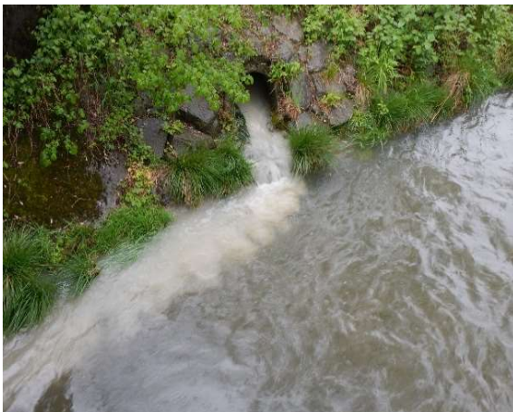
Fig. 1. Combined and separate sewer overflows discharge a wide range of potentially toxic pollutants to surface waters
