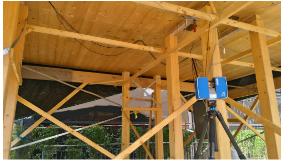
(a) Laser scanner beneath the extrados of the slab
