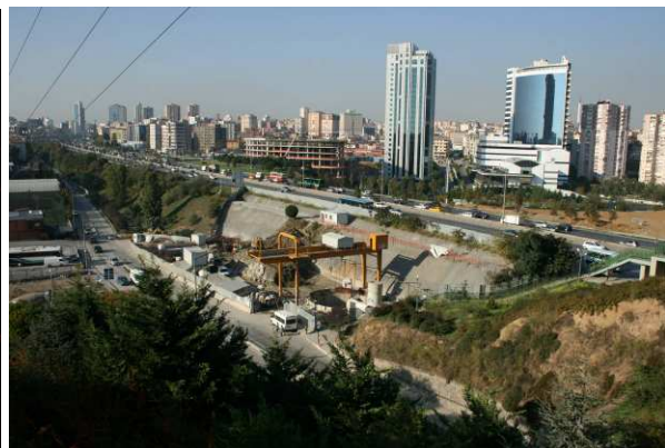
Fig.3.2: A metro worksite along the E5/D100
