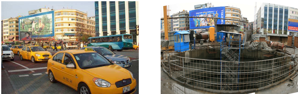
Fig. 7.1: Kadikoy area – interferences between M1-M4 site and facilities at the surface.
