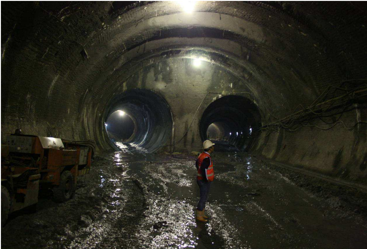
Fig. 7.8: Kadikoy area – M1-M4 complete excavated sections.
