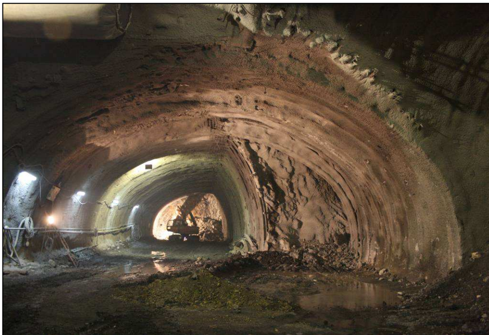
Fig. 7.12: Acibadem station – Excavation inside T type section.
