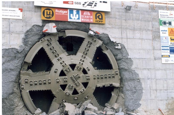
Figure 3. Grauholz 1998 with back-loading cutters
