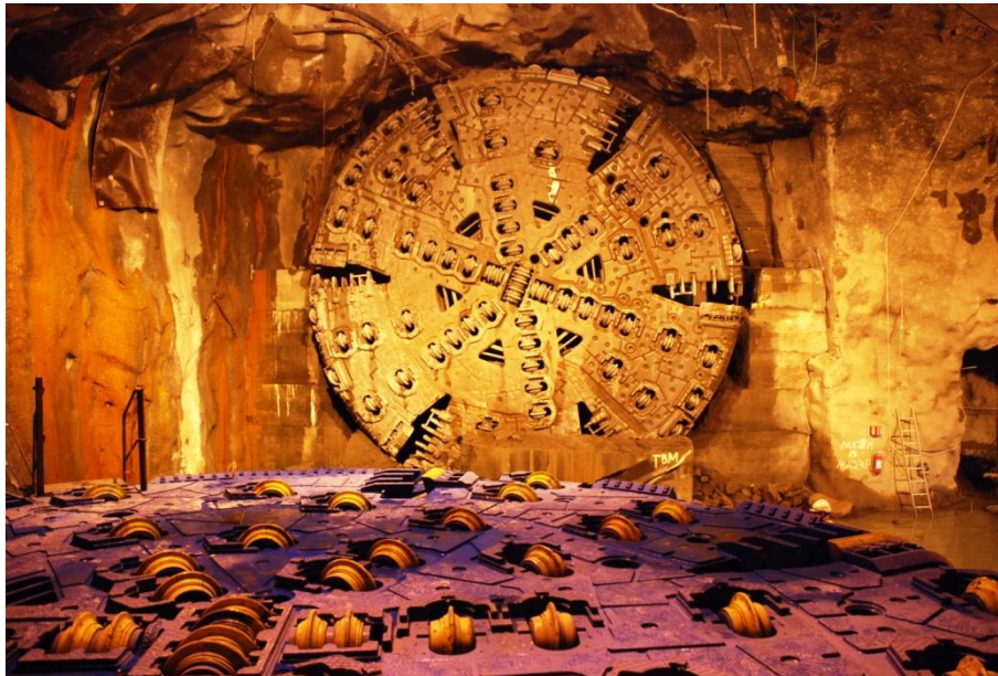
Figure 21: TBM arriving at mid-adit in April 2008 with the second cutterhead waiting in front
