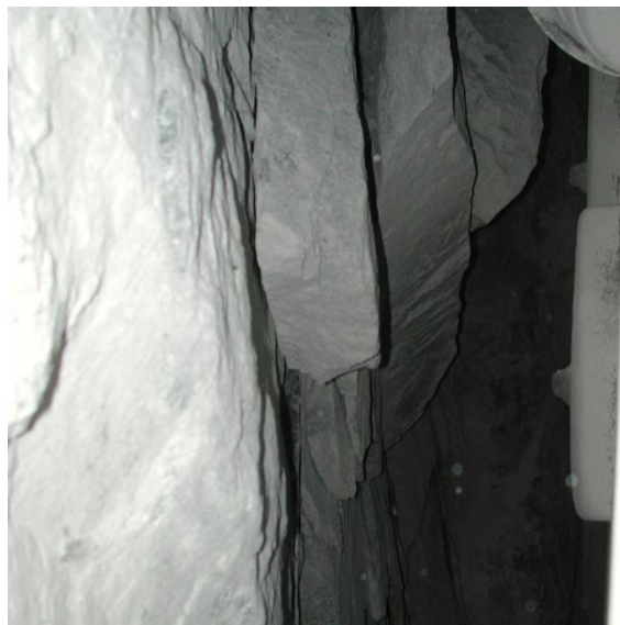
Fig. 10: Lötschberg, blocky face conditions
