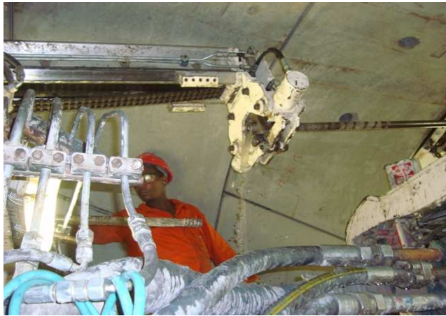
fig. 4a/b: drilling unit, drilling lines / Bohrvorrichtung, Bohrgassen
