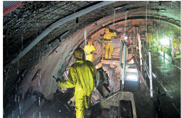
4 Erhöhter Wasserandrang im TBM-Vortrieb Increased amount of ingressing water during TBM drive
