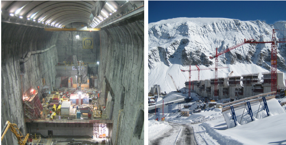
Figure 10. Concreting underway in the machine cavern and at the gravity dam
