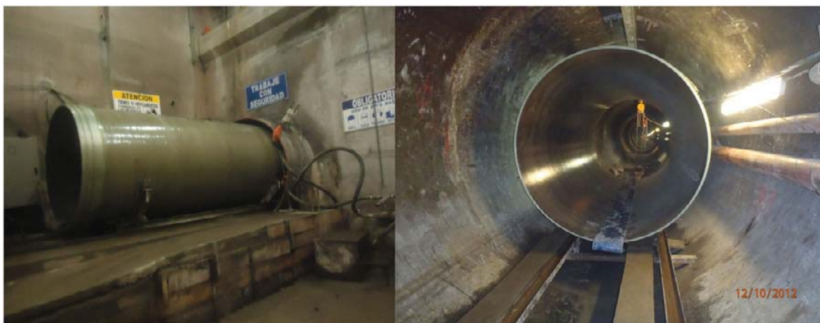
Figure 7. Transportation of pipes to the installation site
