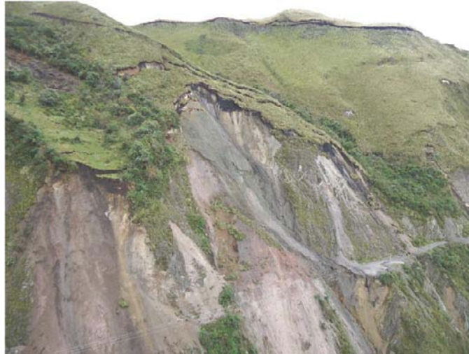
Figure 1. The landslide that affected the headrace tunnel
