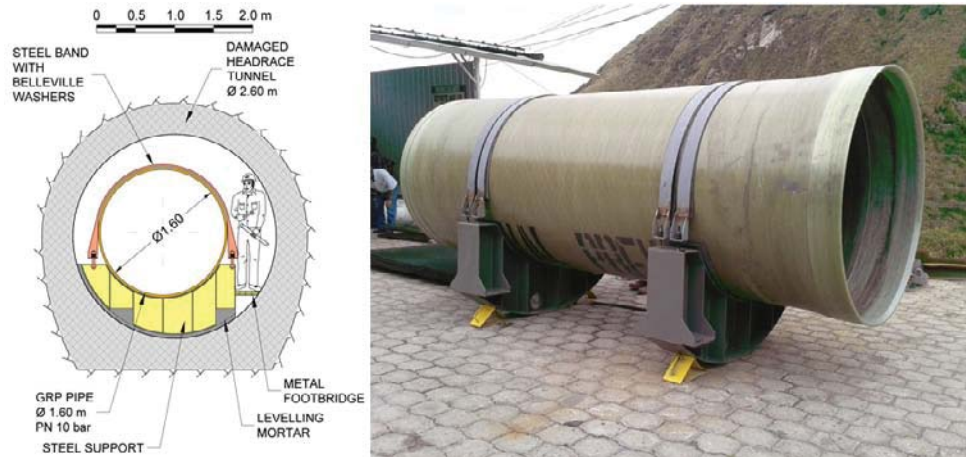
Figure 6. Mounting and adjusting of GRP pipe on steel supports
