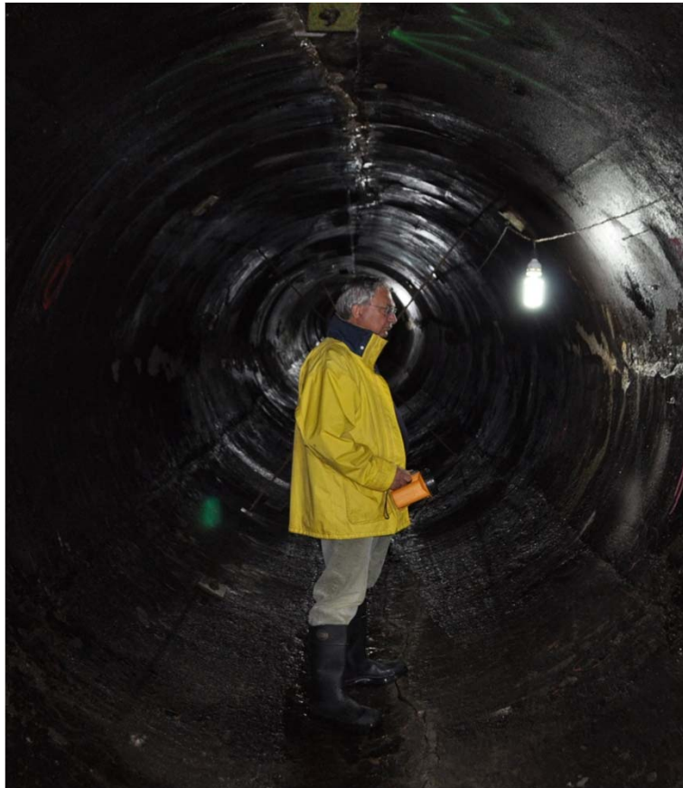
Pucará headrace tunnel in the damaged zone (2011)
