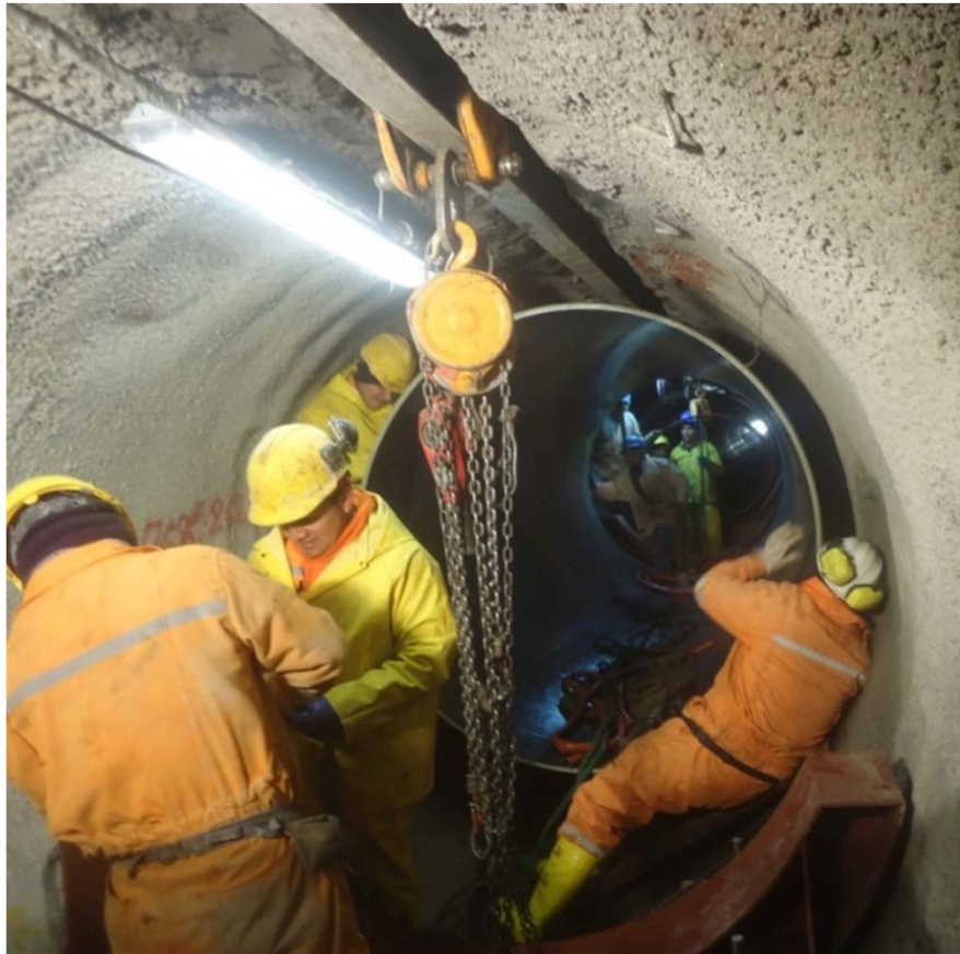
GRP pipe DN1600 in the existing headrace tunnel (D=2.40 m)
