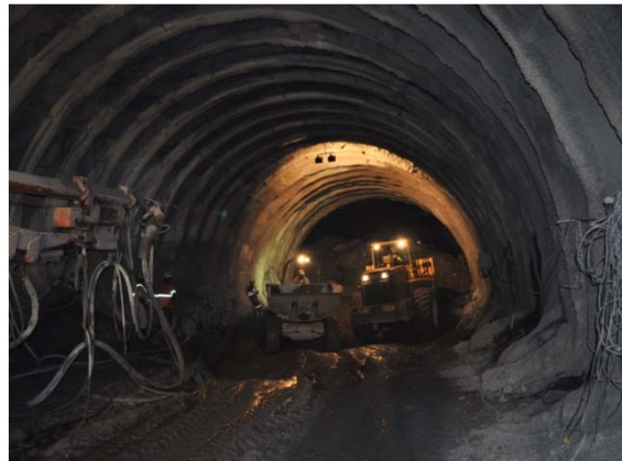
Main collapse crossing works.
