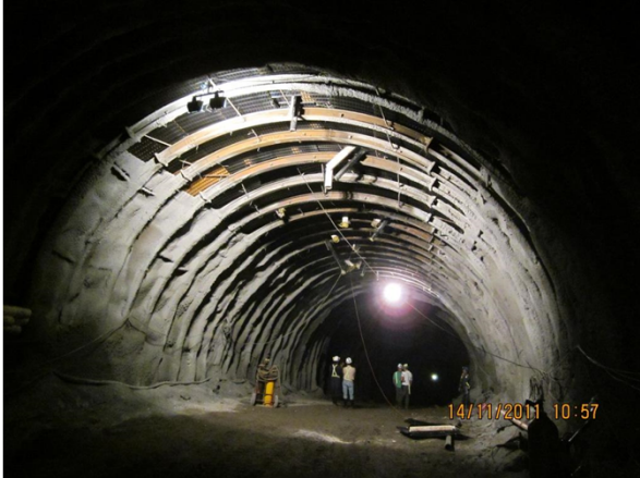
Preparation of the void filling phase with pumped concrete
