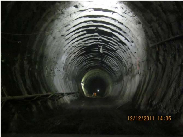
Steel ribs completion phase
