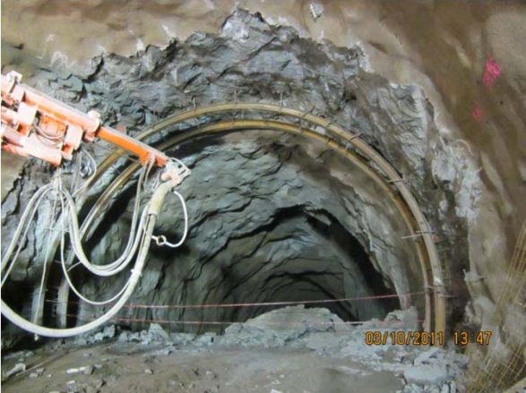
Steel ribs installation phase
