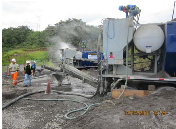
Cement mortar pumping from the surface to partially fill the void.
