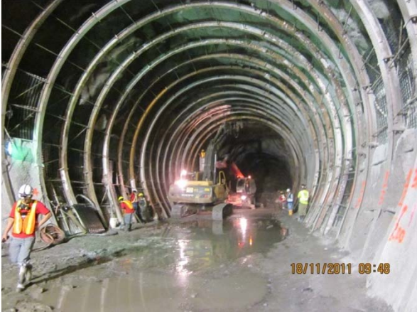
Steel ribs completion phase
