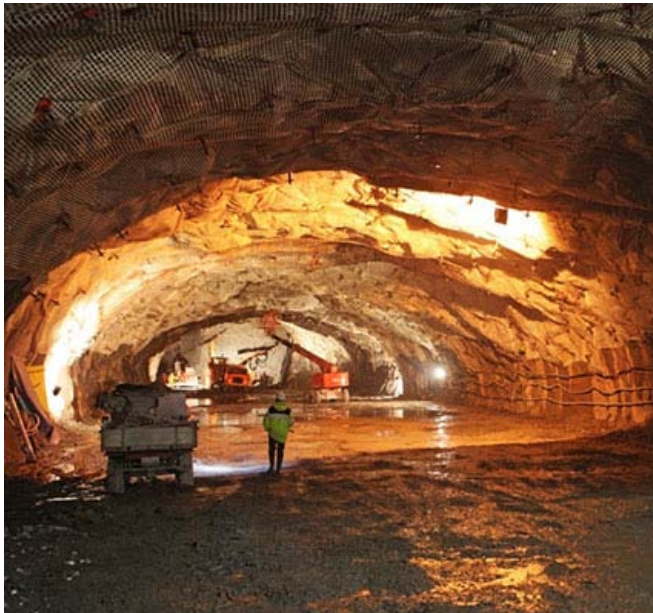
Picture 1 (left) : Powerhouse excavation at stage 1 11 th January 2012 (picture from www.fmhl.ch )
