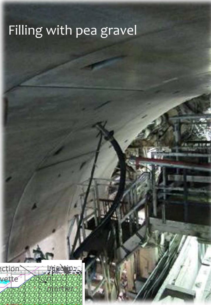
Ring N-2 Filling with pea gravel
