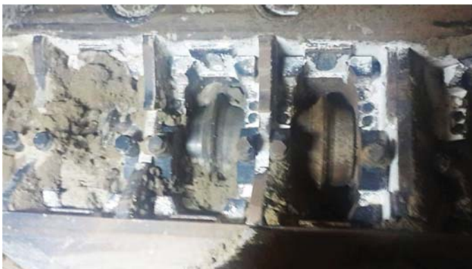
Effect of clogging the cutterhead in Suruc Tunnel
