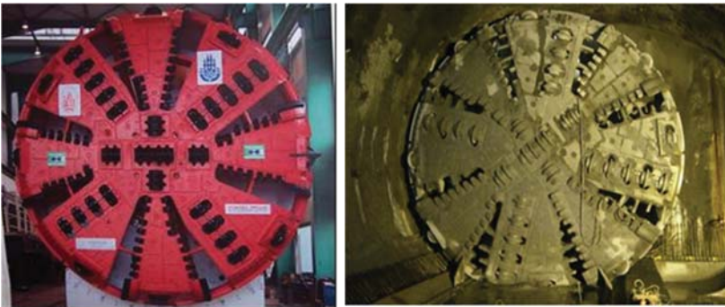
Figure 1-2. Cutterhead before and after modification in Goztepe-Kadikoy Metro Tunnel.
