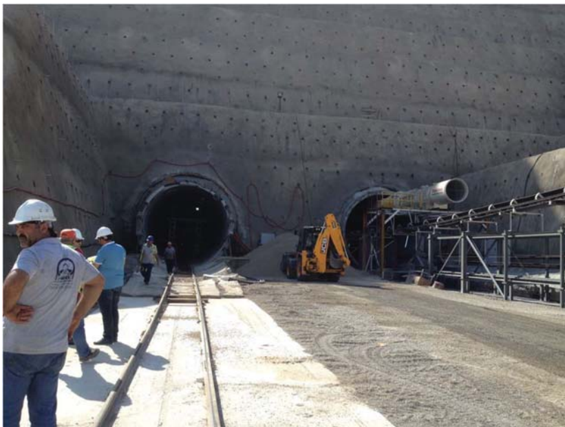
Portal in Nurdağı tunnel
