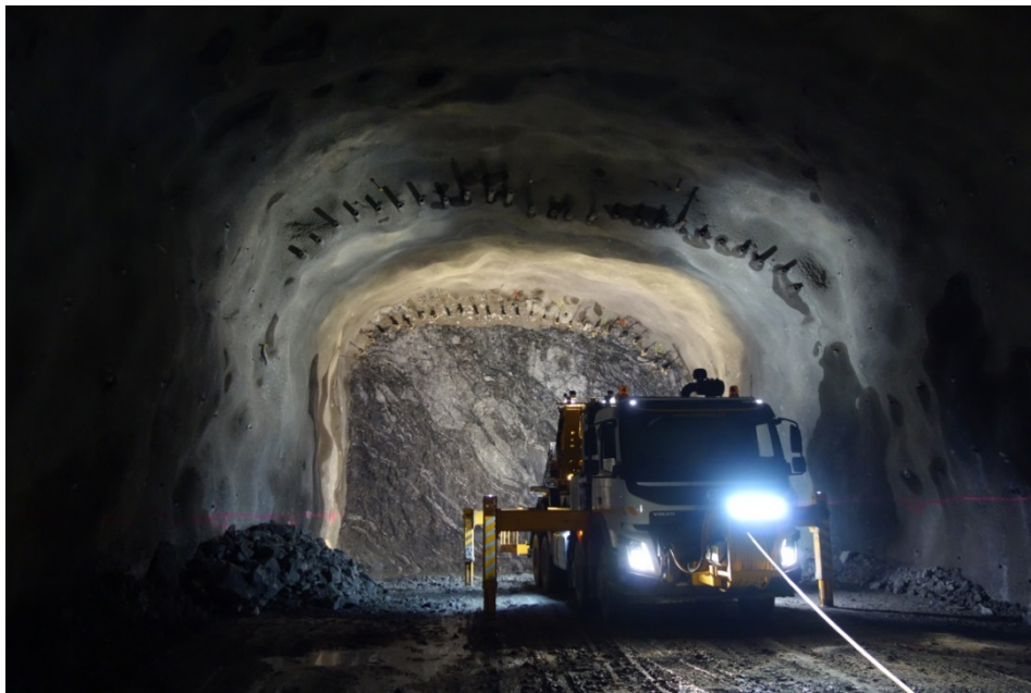
Figure 10. Pipe umbrella and jet grouting in Ramp 412
