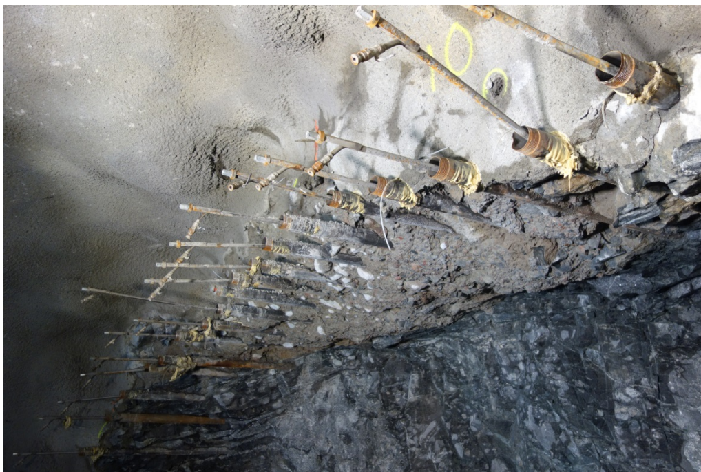
Figure 12. Detail of pipe umbrella and jet grouting
