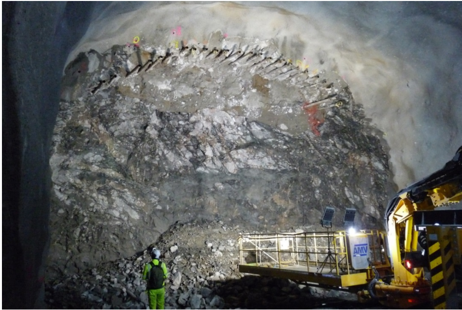
Figure 11. Pipe umbrella and jet grouting in Ramp 411
