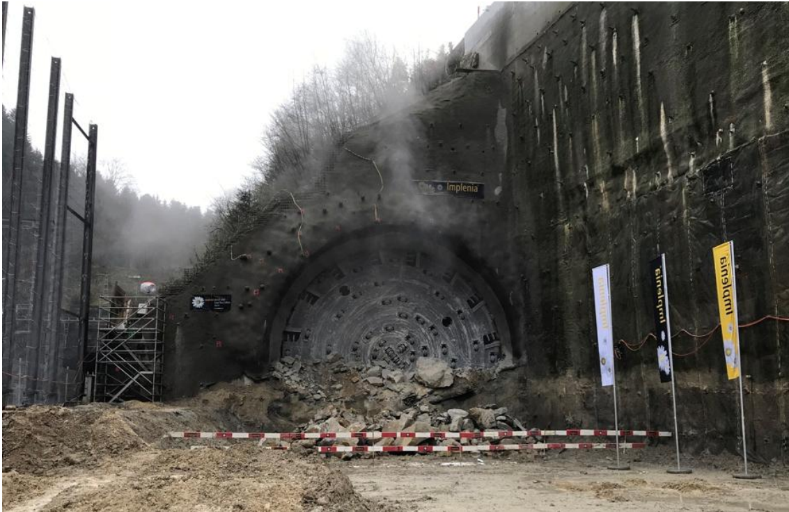
Figure 8. TBM break-through.
