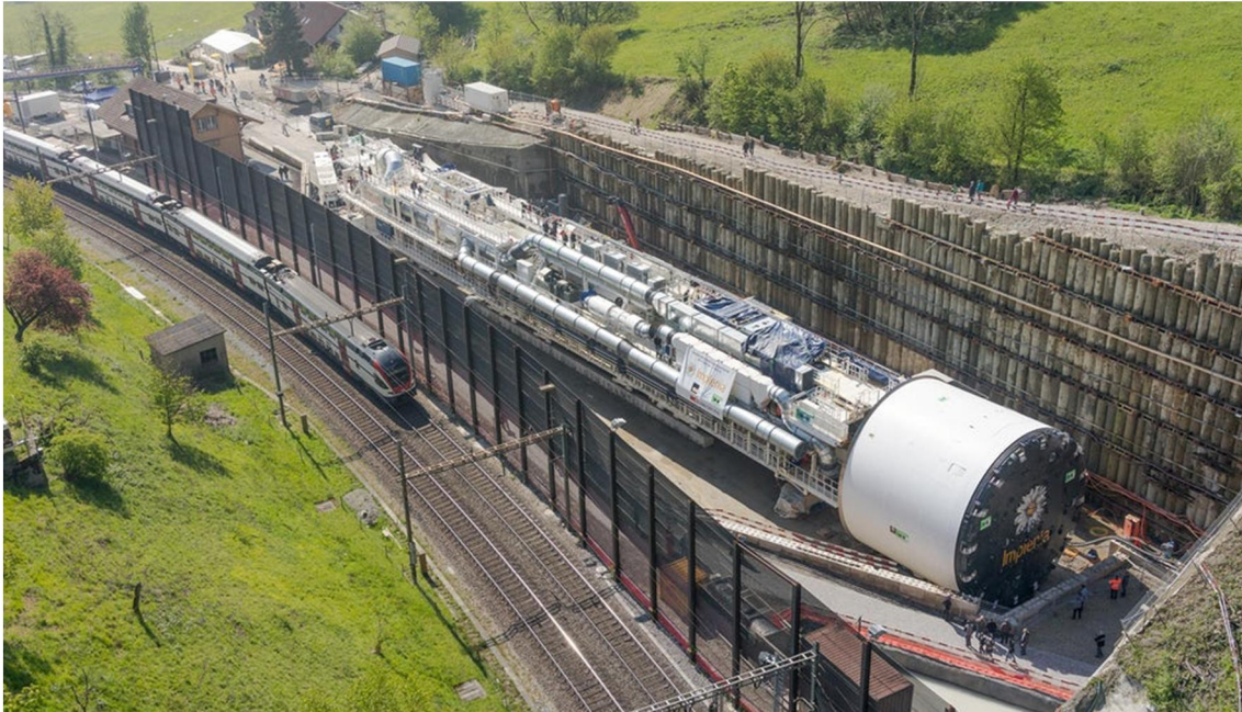
Figur 4: Herrenknecht single shielded TBM, Ø 12.36 m (picture: courtesy of Swiss Federal Railways).
