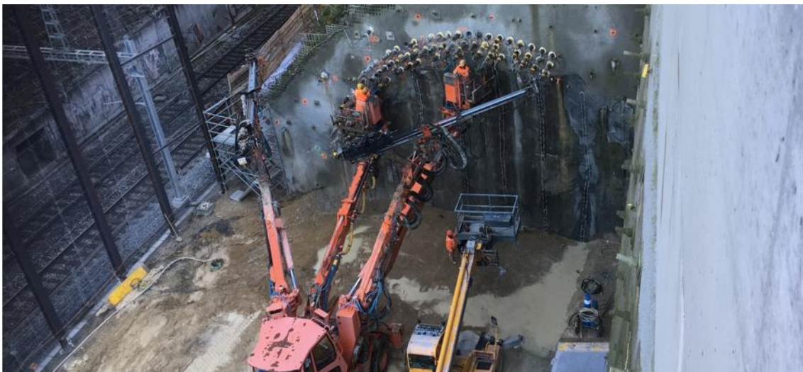
Figure 11. Installation of the triple pipe umbrella (picture: courtesy of Implenia Switzerland).
