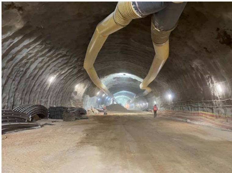
68 | 18.11.2021 | Road 60 tunnels, Israel
