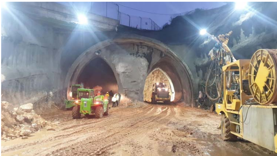
52 | 18.11.2021 | Road 60 tunnels, Israel
