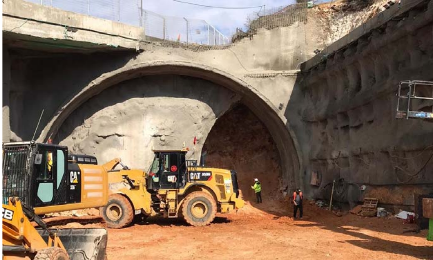
51 | 18.11.2021 | Road 60 tunnels, Israel
