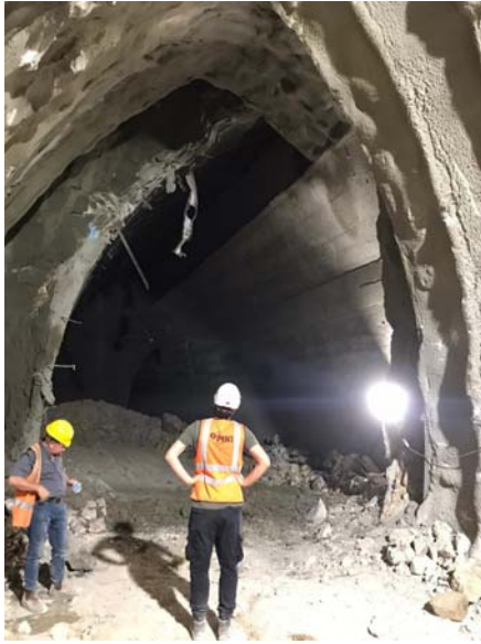
67 | 18.11.2021 | Road 60 tunnels, Israel
