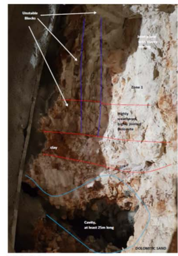
Fig. 4. Hebron (left) wall
