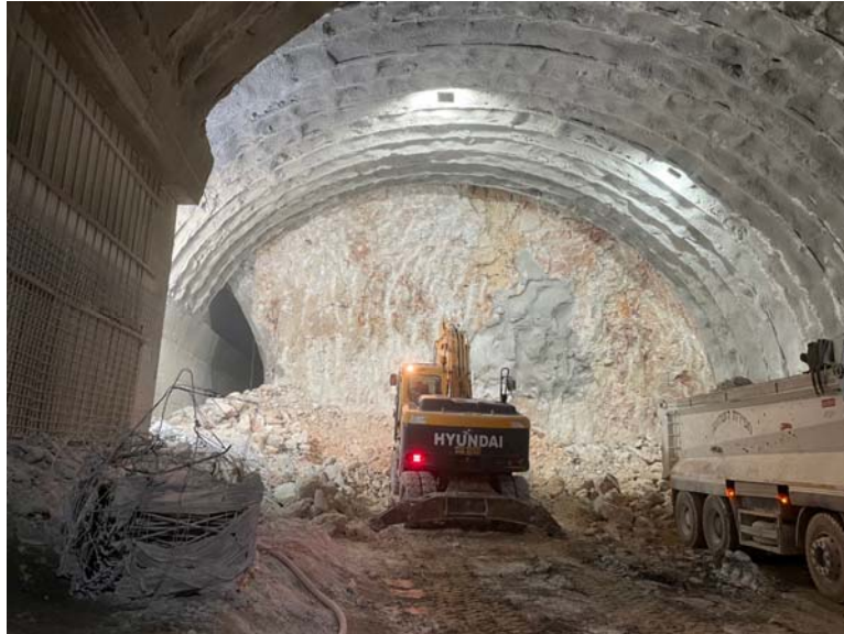
69 | 18.11.2021 | Road 60 tunnels, Israel
