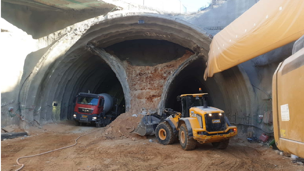
53 | 18.11.2021 | Road 60 tunnels, Israel
