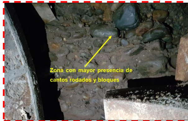
Face condition TBM tunnel
