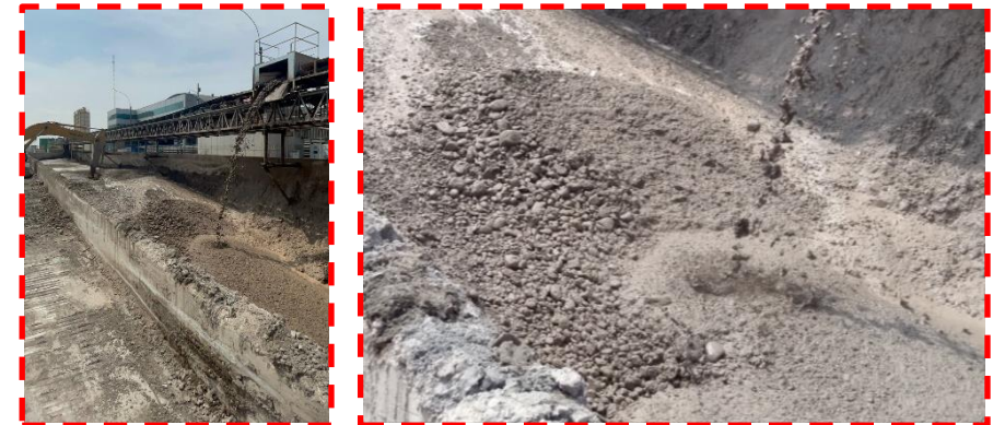
Soil condition after TBM excavation
