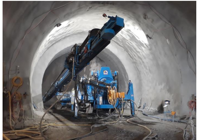
Figure 7. jet-grouting operation
