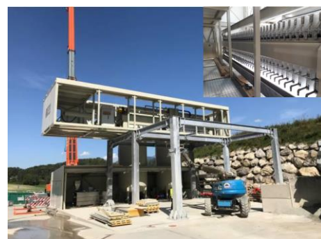
Figure 8. construction of the sludge filter press
