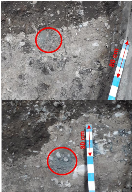
Figure 9. Observation of the face columns (small diameter on the top, good diameter on the bottom)
