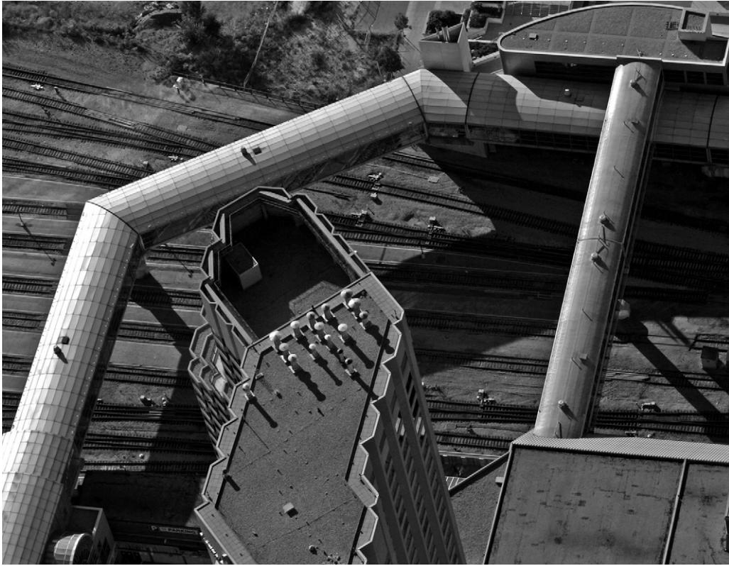
Fig. 7. Hybridized network: low-altitude aerial view of the skywalk passing over the regional train corridor in downtown Toronto, 2004.
