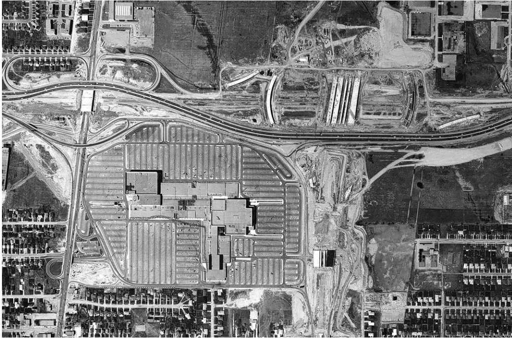
Fig. 5. Construction of the Yorkdale Shopping Mall on the northern periphery of the Greater Toronto Area, 1964. Source: Sanborne Aerial Imagery.
