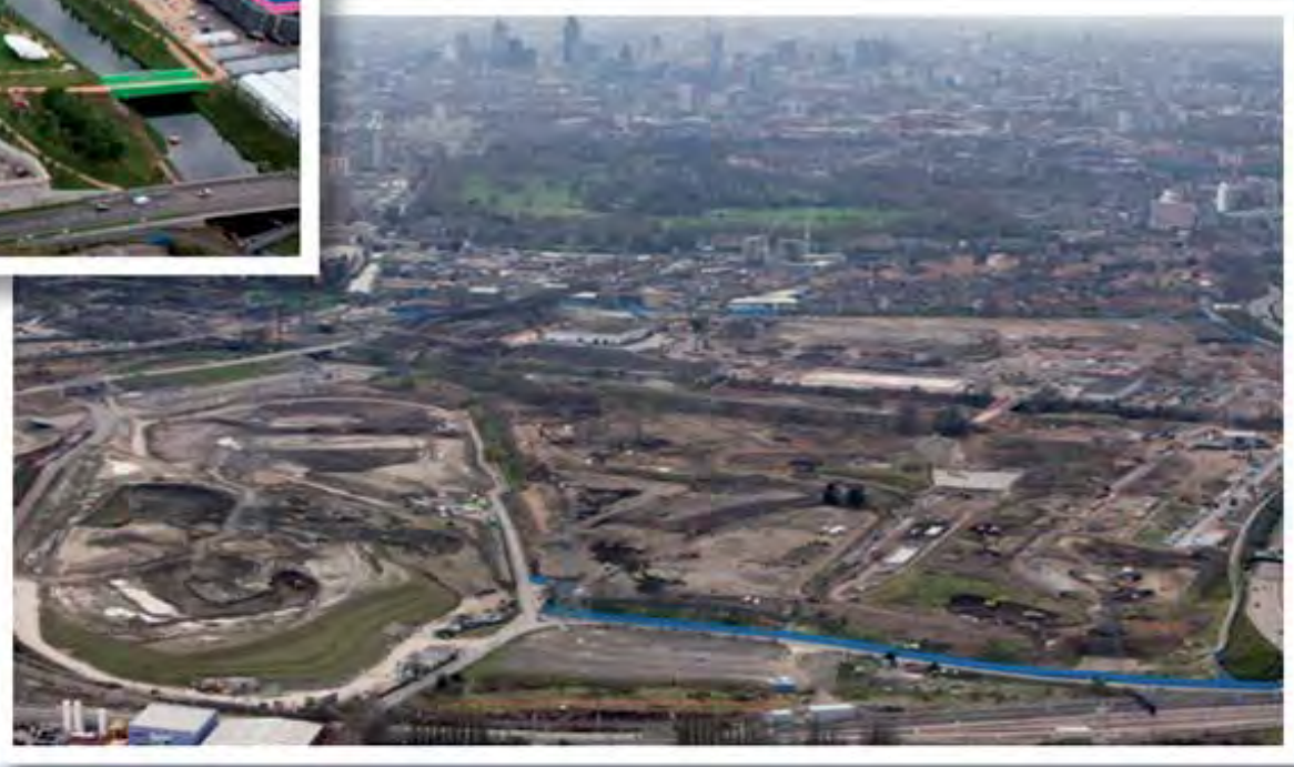
Source: Olympic Delivery Authority. 2012 photograph looks South from Eton Manor. 2008 photograph
