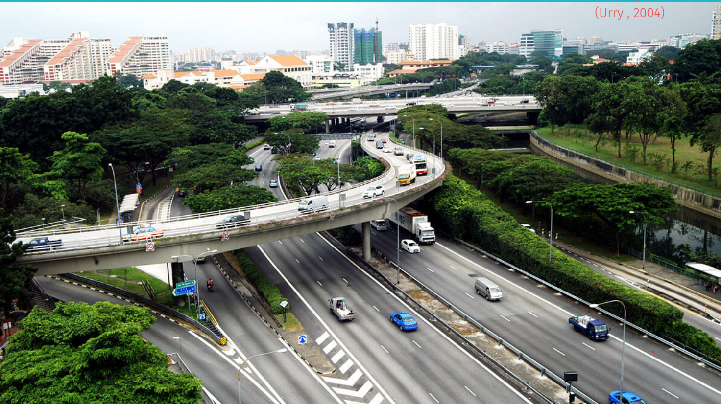
View of a highway in Singapore
