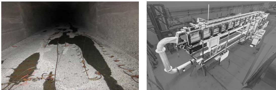
Abb. 4: (a) Invert abrasion of Asahi SBT in Japan: several decimeter-deep incision channels of the reinforced concrete (Müller-Hagmann, 2017) (b) Experimental flume, small-scale SBT model at VAW (Photo: VAW, ETH Zurich).
