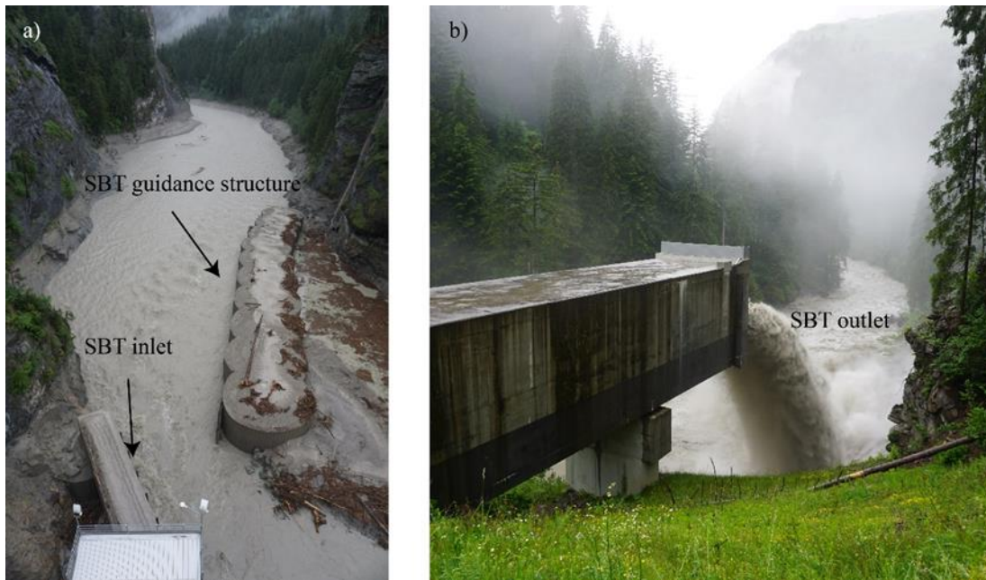
Fig. 4 Photos from Solis Sediment Bypass Tunnel inlet (a) and outlet (b) in operation during a five-year flood event on 12 th June, 2019 (photos: I. Albayrak, VAW).
